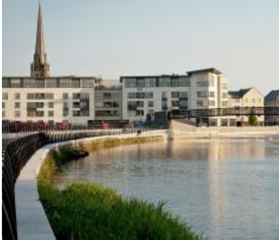
Flood defence wall along east bank of River Barrow
