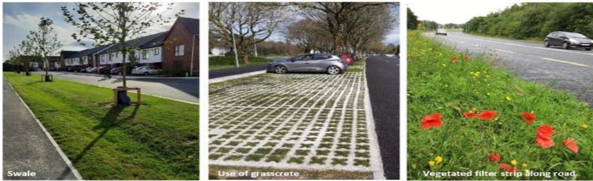
Fig. 7.3: Examples of SuDS (Source: DHLGH ‘Nature-based Solutions to the Management of Rainwater and Surface Water Runoff in Urban Areas – Best Practice Interim Guidance Document, 2022’)
