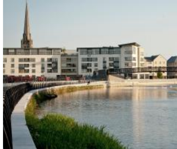
Flood defence wall along east bank of River Barrow
