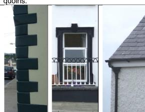
Building features: chamfered, faux quoins; raised plasterwork window surround with keystone detail and wrought iron railings to front; natural slate roof and caste iron hopper
