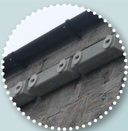
Double nest-cavity Schwegler Swift nest boxes installed at Mullingar Courthouse
