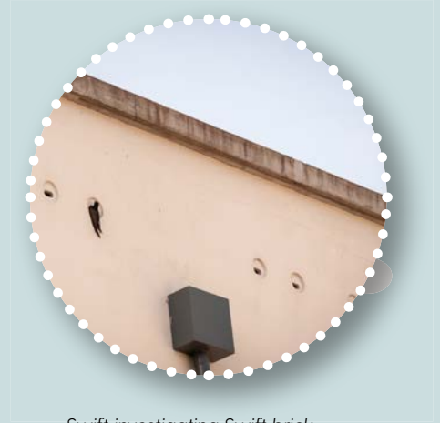
Swift investigating Swift brick nest boxes at Westport Town Hall
