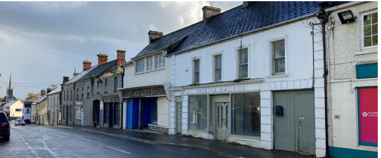
Vacant and derelict buildings along Main Street
