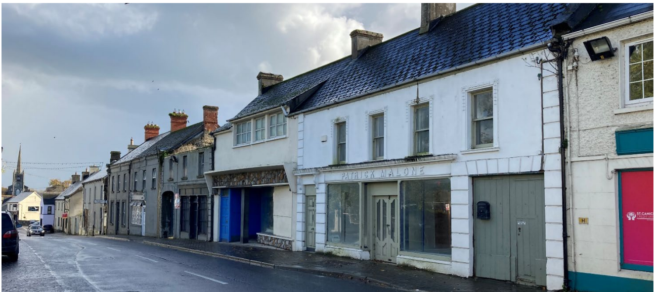
Vacant and Derelict Properties along Main Street
