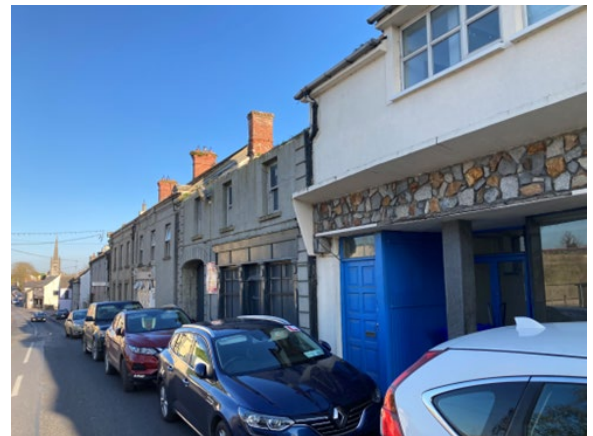
Derelict heritage building
