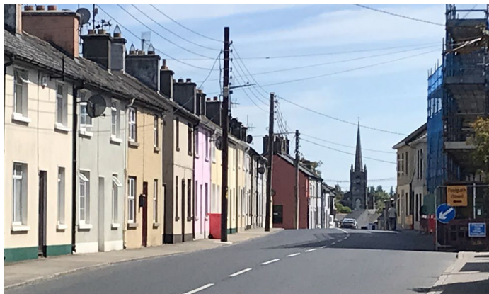
Overhead cables, Main Street
