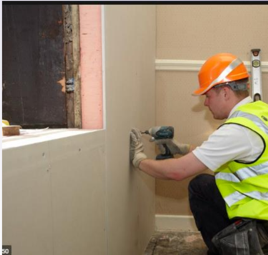
Internal insulation
