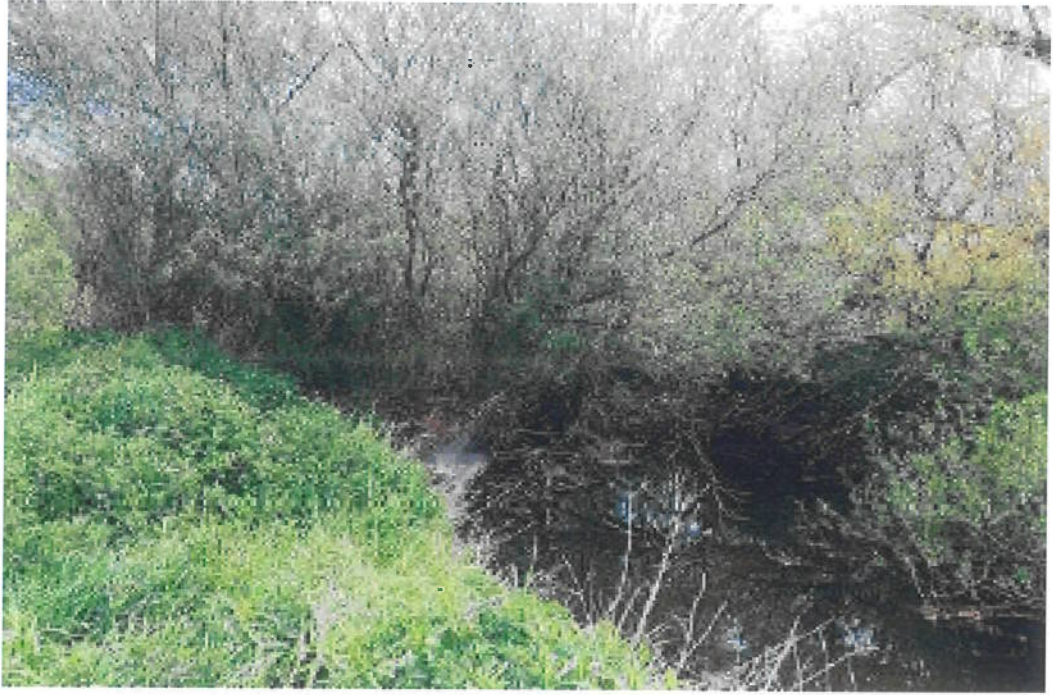
Stradbally River (trees encroaching into river and fallen trees) ~ Before
