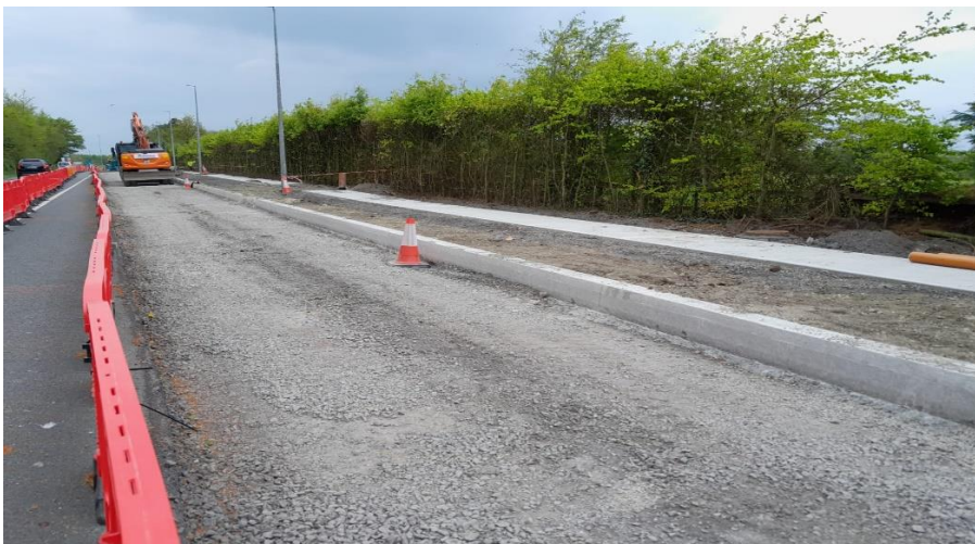
N77 Abbeyleix Road Pavement, Safety & Active travel scheme progressing to programme.
