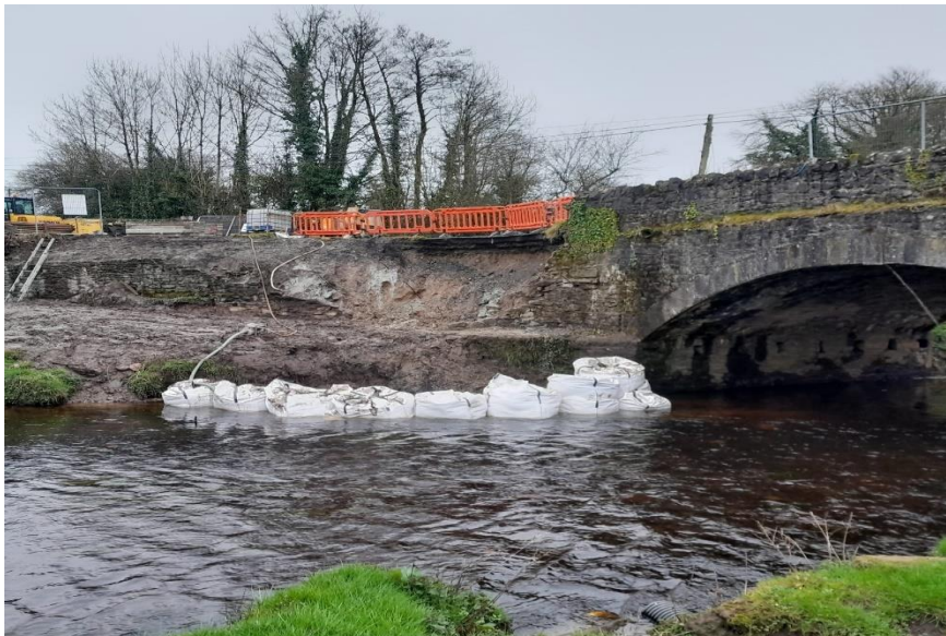
Emergency bridge repairs ongoing on Forest Bridge following retaining wall collapse
