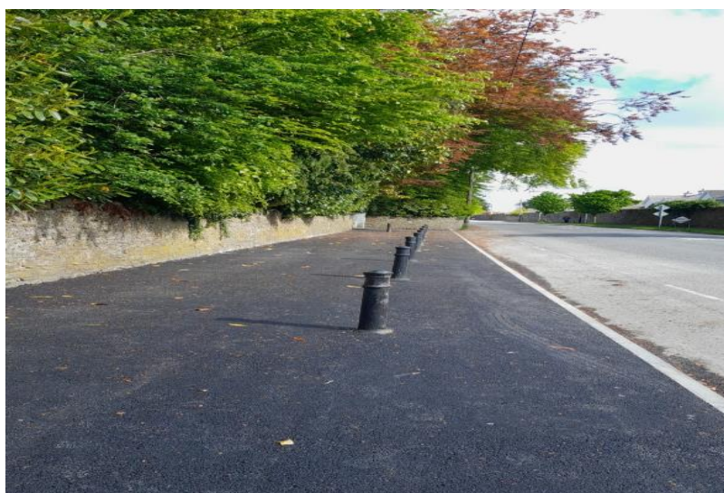
Completed footpath works in Ballyroan in advance of Restoration Improvement works.
