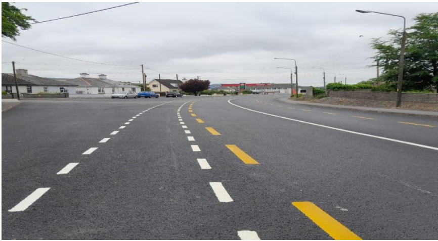
Recently completed road strengthening works on the R639 Durrow
