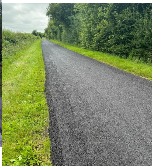
Micro-surfacing Ballyfin
