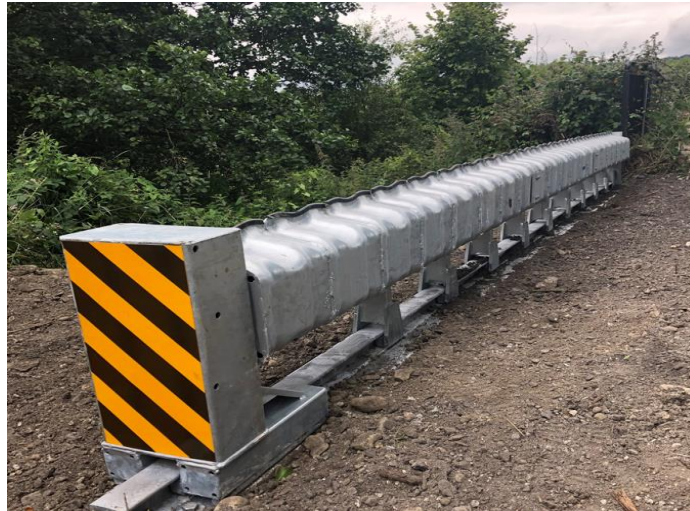
New vehicle restraint barriers installed on the L-7894-0 at The Strand
