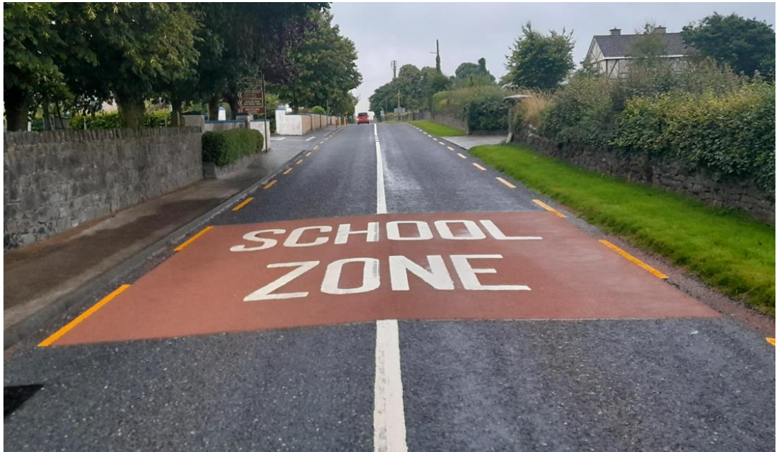
Tintore to Ballacolla Restoration Improvement Works
