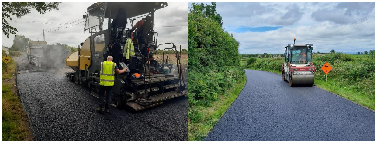
Road strengthening works at Clonreher & Tullore
