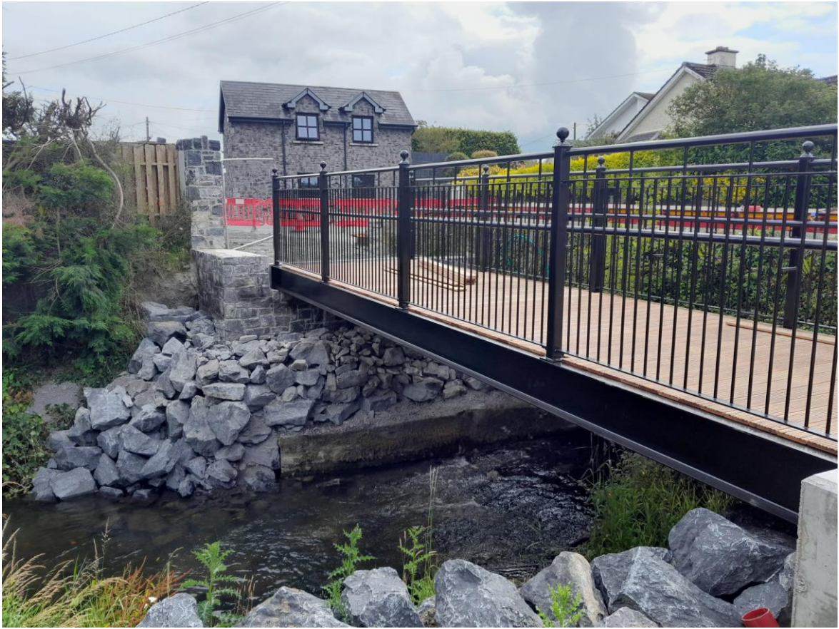
Junction Improvements & Pedestrian Bridge installation Green Mill Lane
