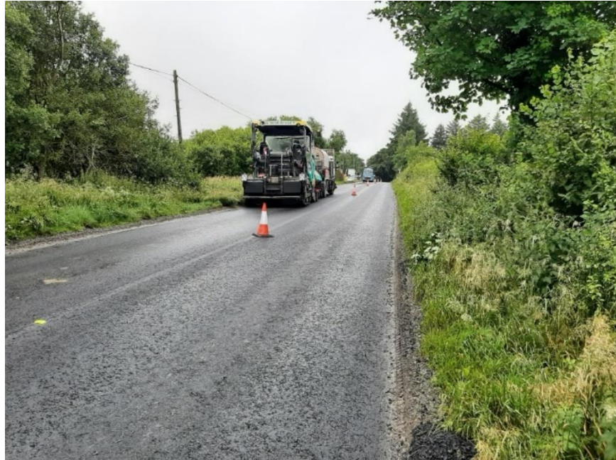
N78 Ballylehane Lower to Farnans works ongoing.
