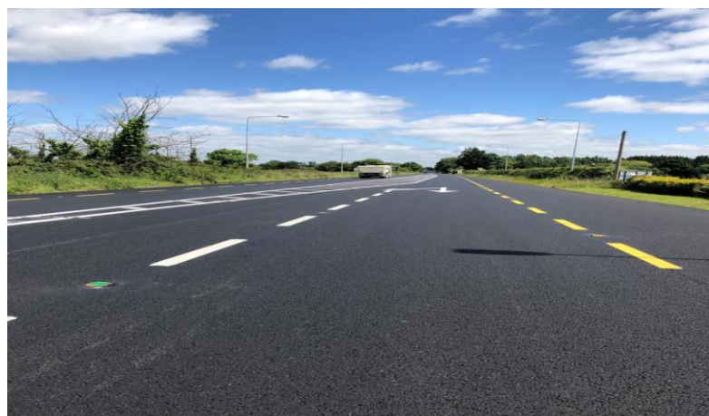
Resurfacing Works Completed on R445 (Former N7)
