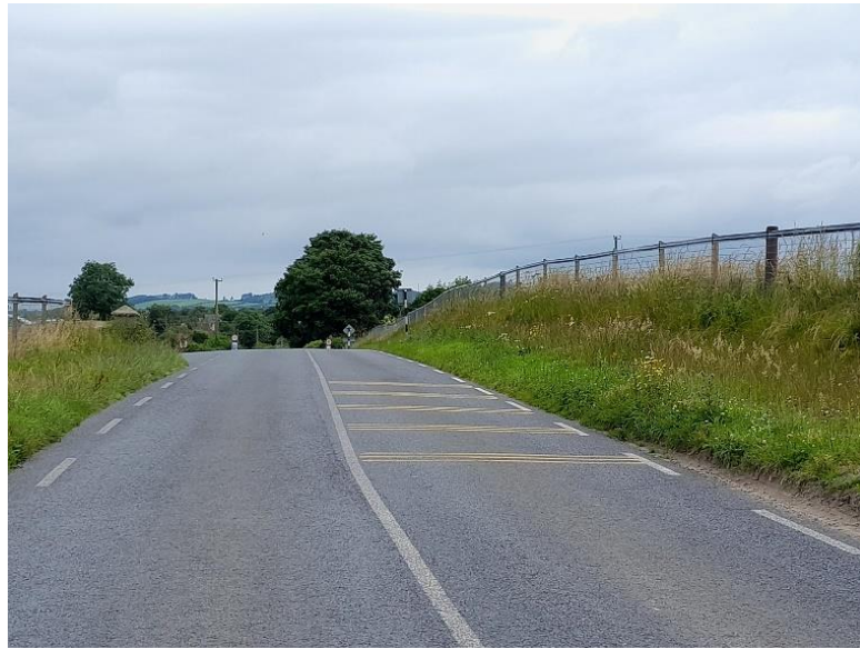
Safety Improvement works at R425 Ballyroan Rd, Abbeyleix
