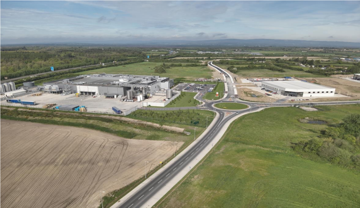
J17 National Enterprise Park Western Arm works progressing towards completion
