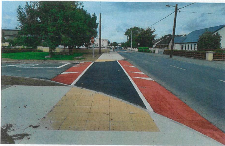
Junction tightening and raised uncontrolled crossing
