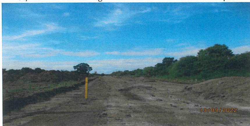
J17 Access Road looking North towards Iarnróid Eireann Depot
