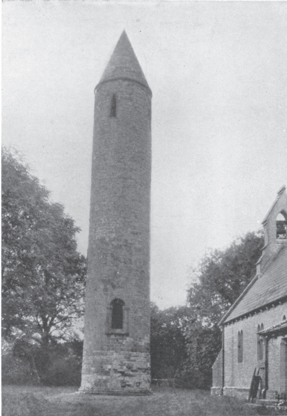
TIMAHOE ROUND TOWER. (The East Side, showing how the Tower leans.)
