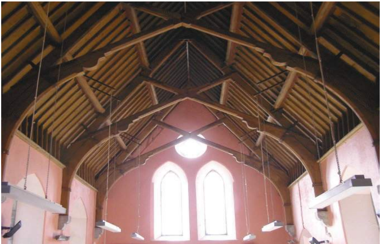
Figure 20: Interior of former church
