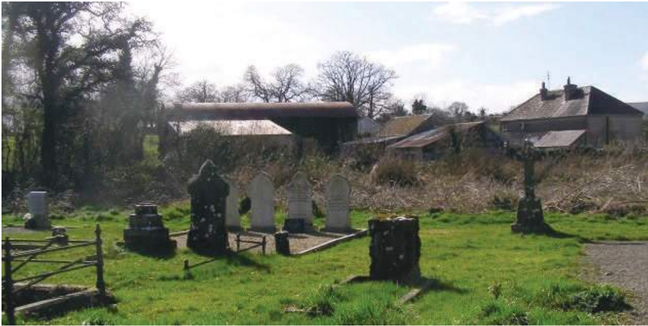
Figure 16: Scrub and decaying vegetation on site
