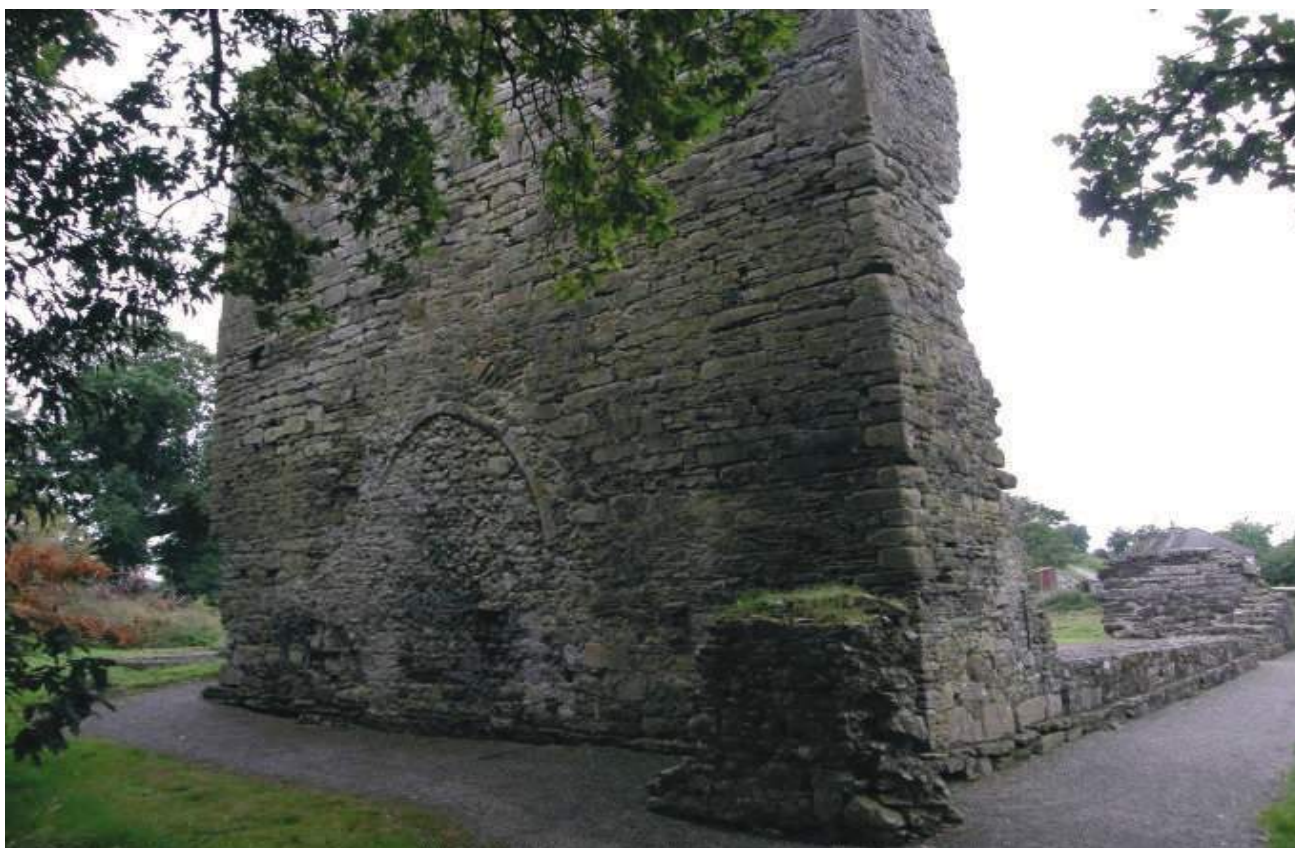
Figure 8: Gable of church/castle with blocked arch
