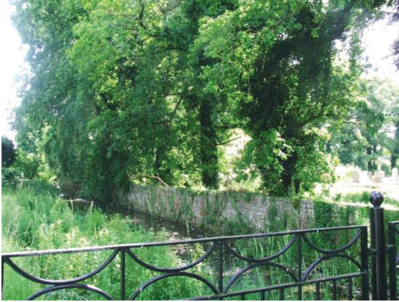
Fig. 10: The Timahoe river and its associated fringe of vegetation at the eastern entrance to the site
