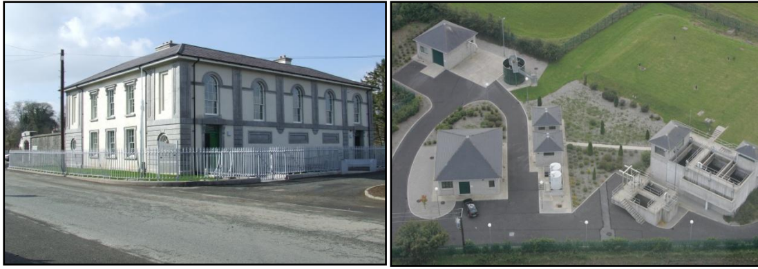
Stradbally Courthouse and Arts Centre [left] and Ridge Road, Portlaoise Treatment Plant [right]
