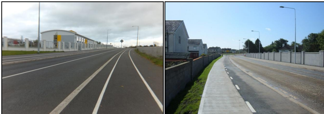
Portlaoise: section of SOR with new schools campus [left] section of WOR at Clonrooske [right]
