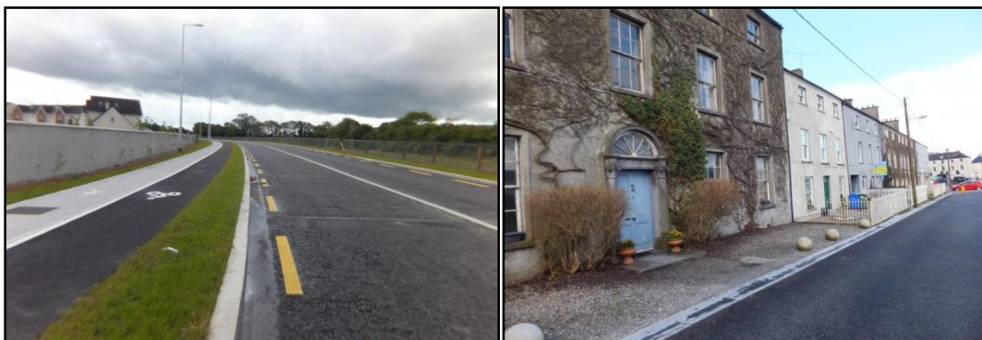
Carlow: extended section of Northern Relief Road [left] and Durrow Square refurbishment [right]
