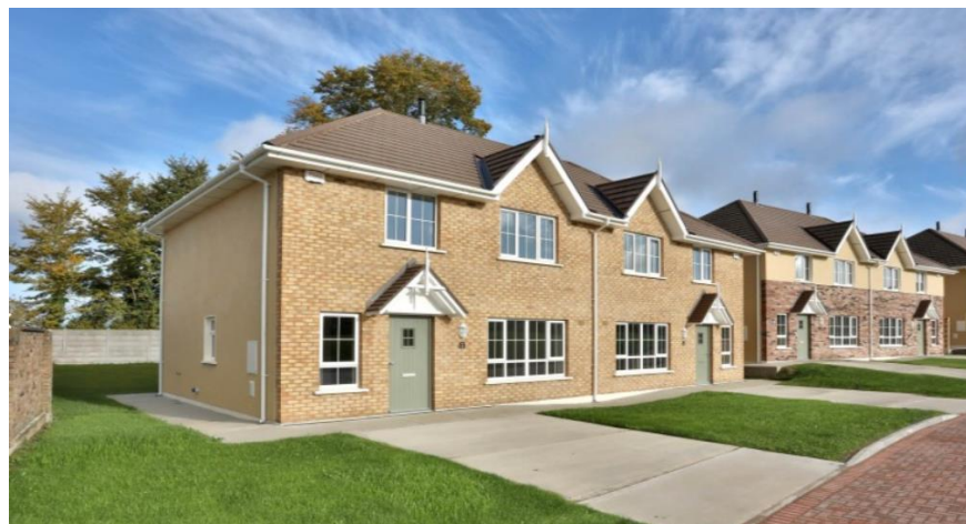
Plate 7: New housing at Maryborough Village, Mountrath Road
