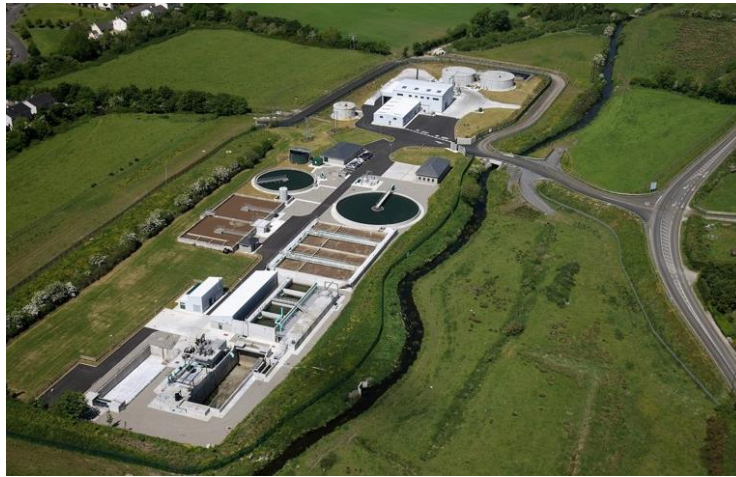
Plate 12: Uisce Eireann Treatment Plant at Ridge Road
